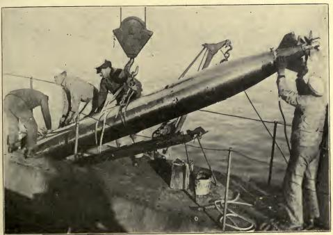
MANEUVERING TO LOAD THE TORPEDO INTO ITS TUBE
