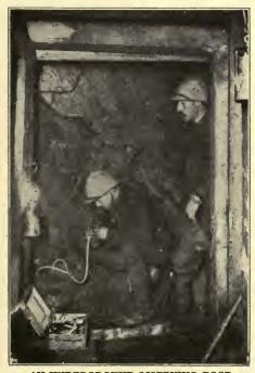
AN UNDERGROUND LISTENING POST Listeners in branch galleries sometimes used stethoscopes to catch the faintest sound indicating an attempt at a counter-mine by the enemy.
